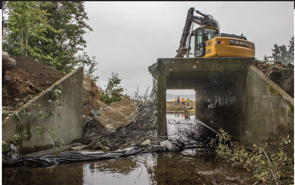
A box culvert is removed in August 2014 to improve fish passage at the mouth of Chico Creek.
